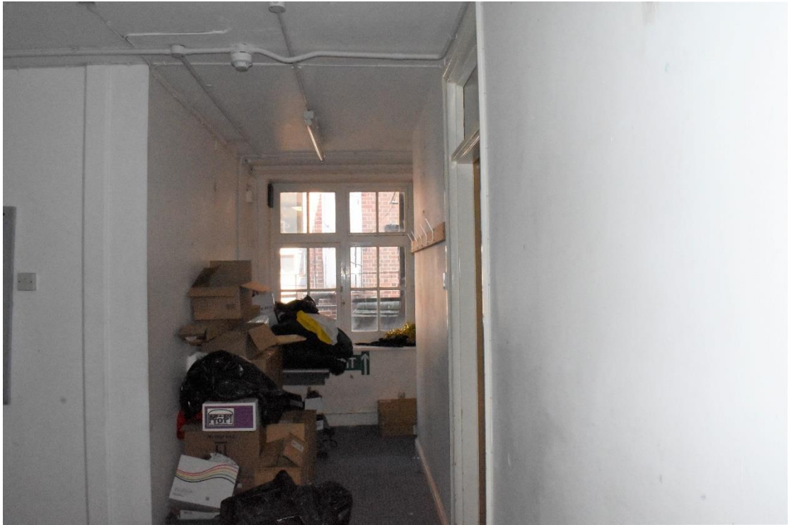
Plate 26. View of the current first floor fire exit, not in use, note the ledge to climb up (looking W)
