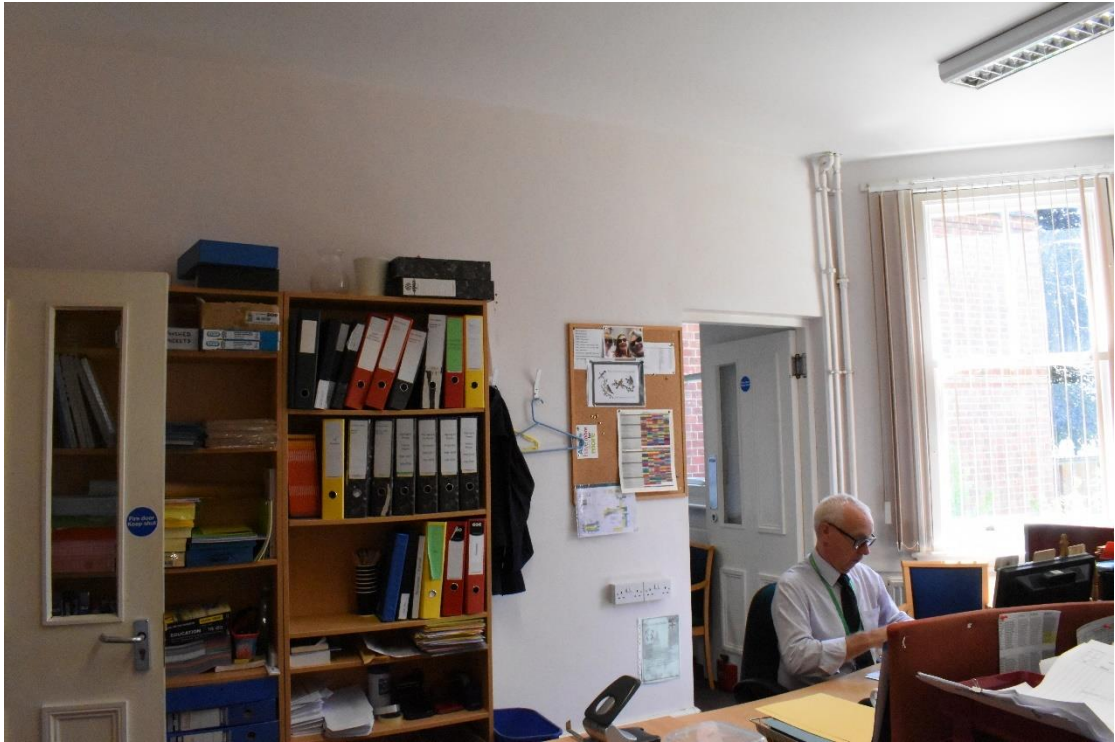
Plate 16. View of the wall between the Easternmost offices to be removed (looking SE)
