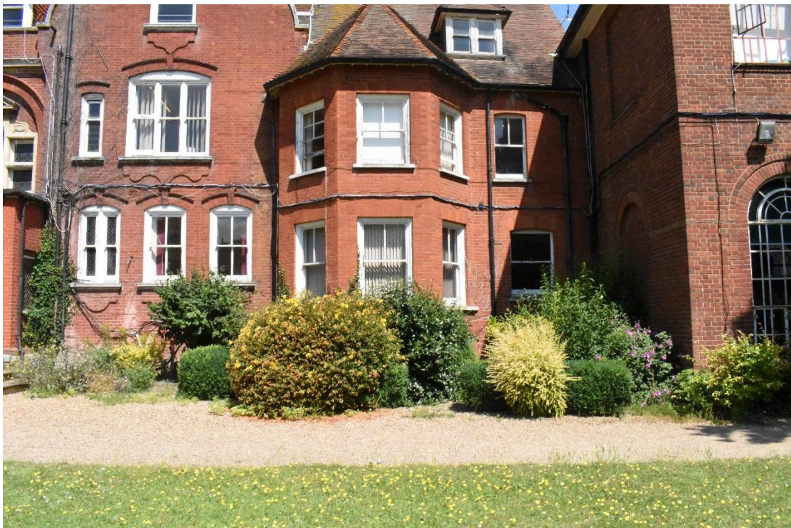
Plate 12. View of the ground floor windows (looking NNW)
