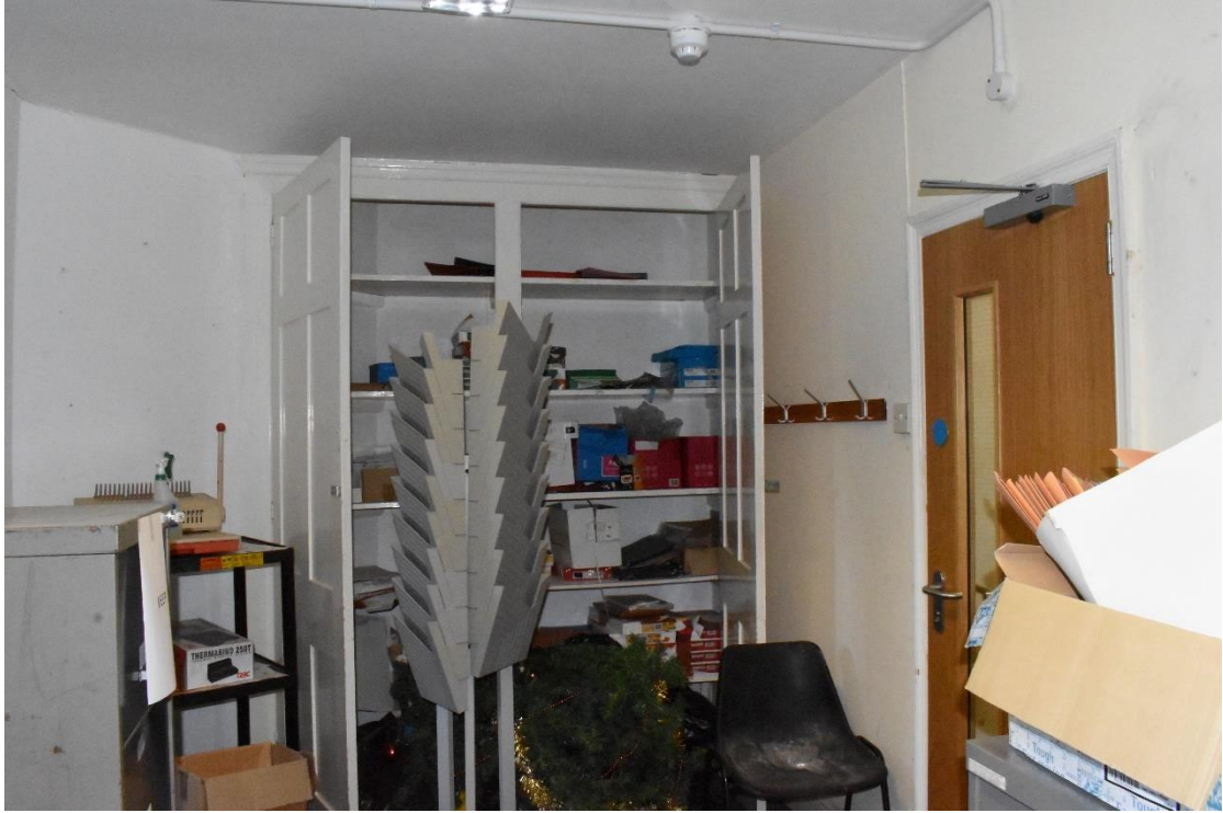
Plate 31. Internal View of the wall in the southern room that will be removed (looking NNW)
