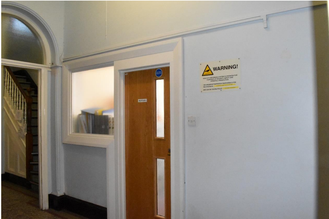
Plate 14. Entrance to Bursar's Office – to be blocked up (looking SE)
