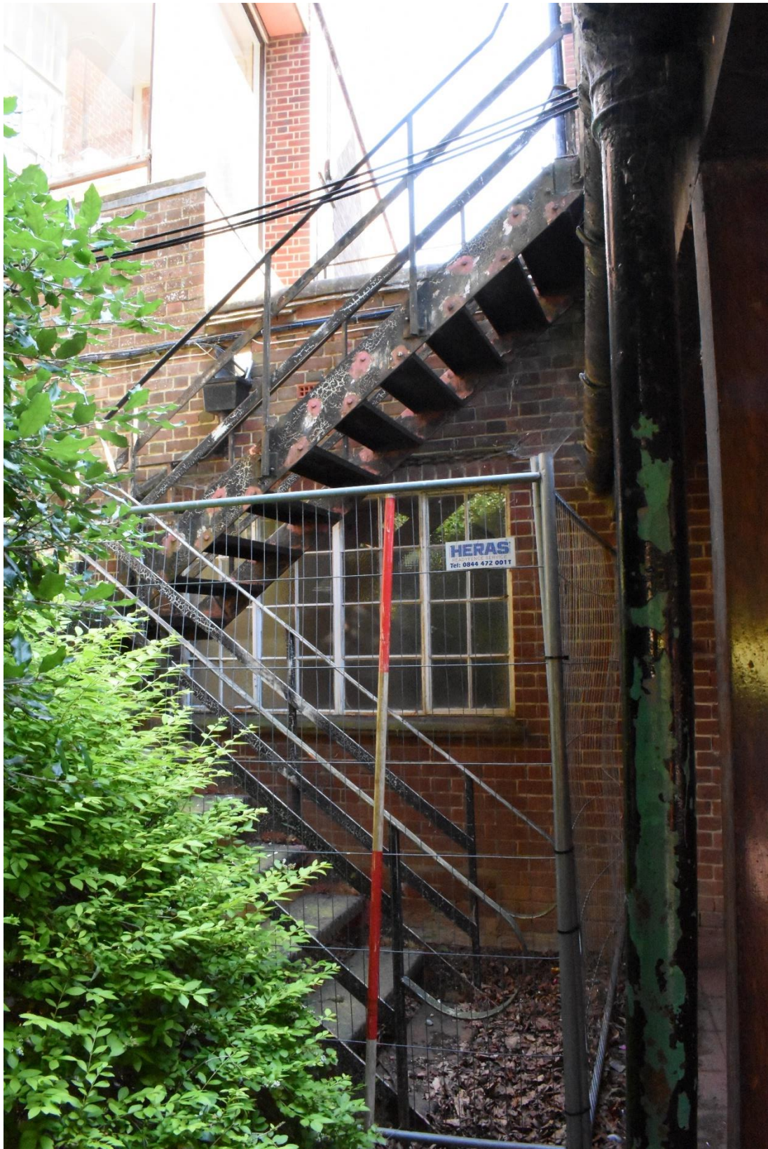
Plate 27. External view of the current fire escape from the ground floor (looking ENE)
