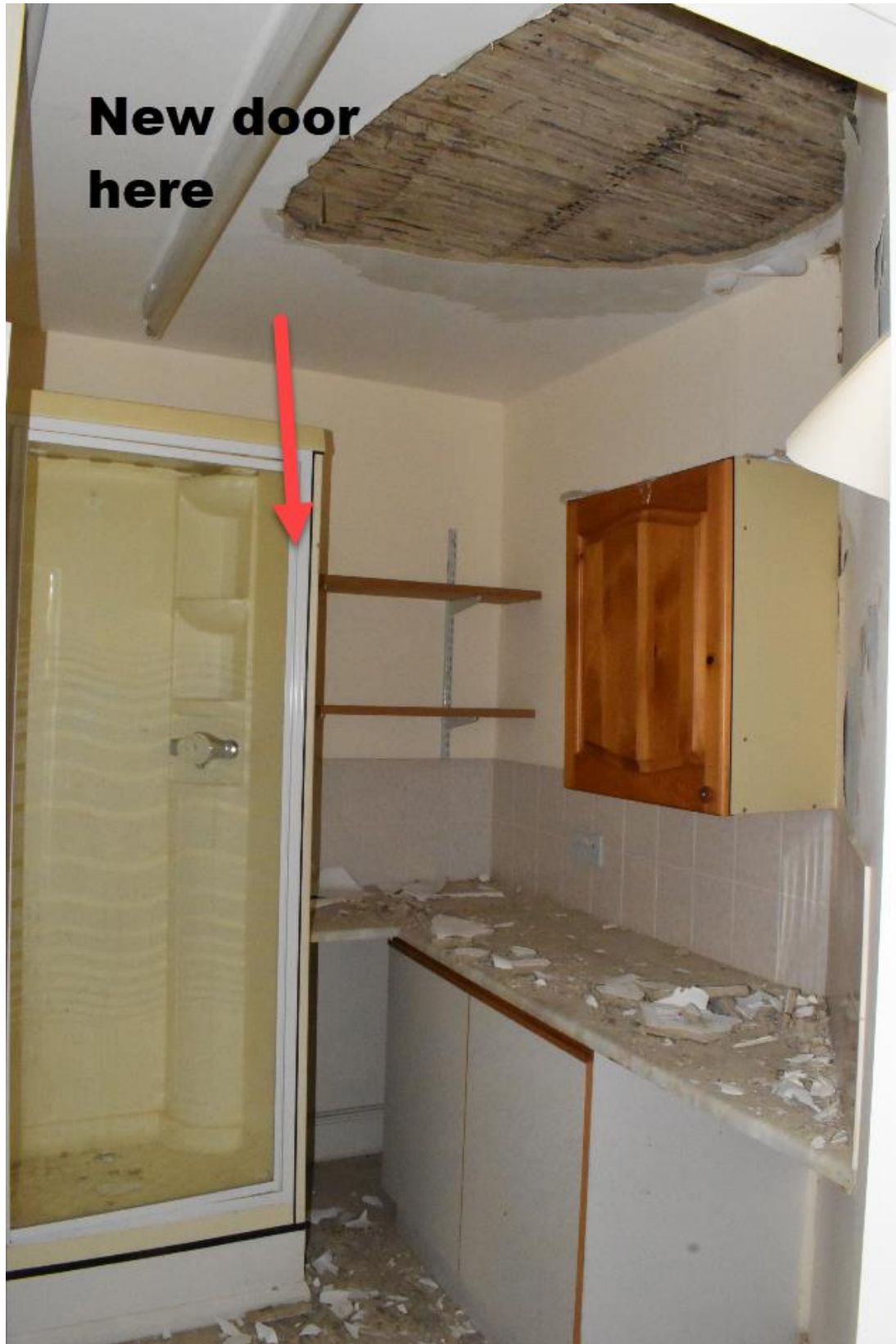
Plate 30. Internal room view of the wall for the new door (looking W)
