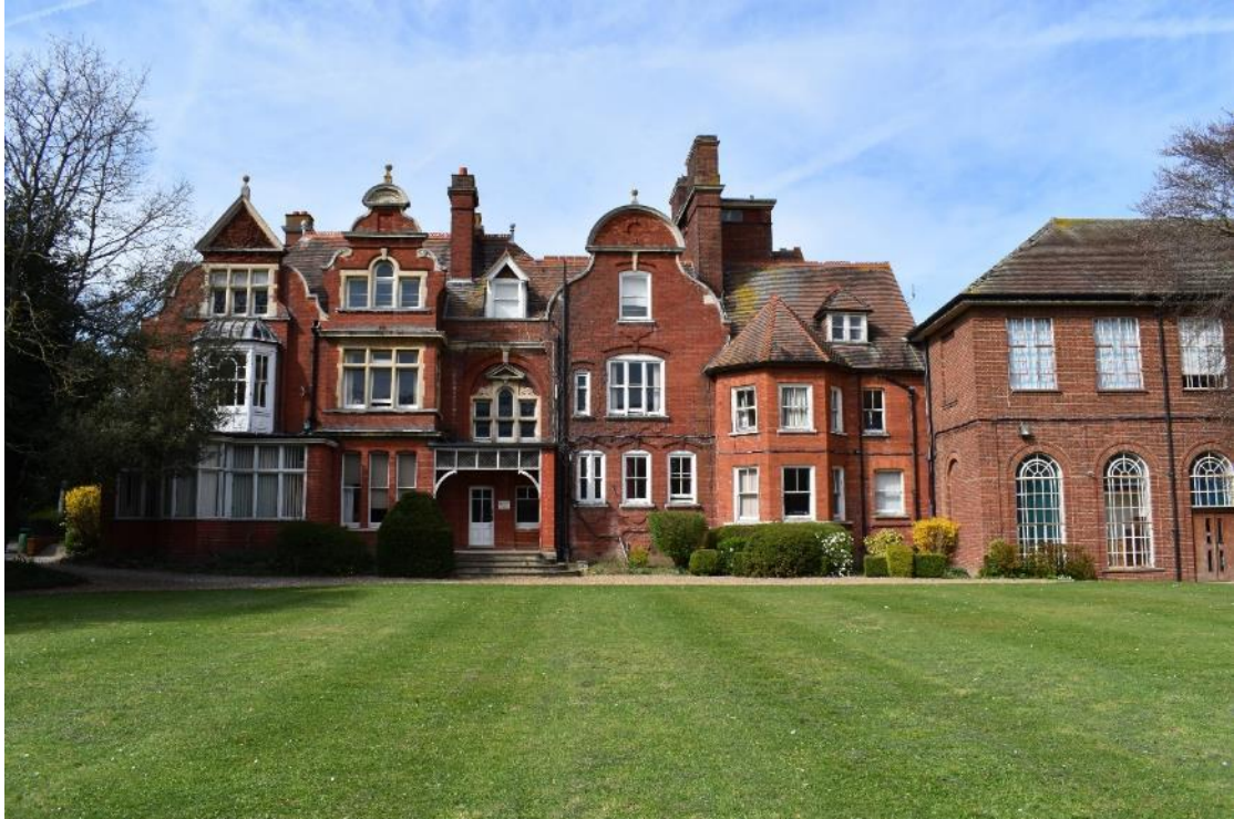
Plate 9: Rear of Hatton House (facing NNE). Scale 2m
