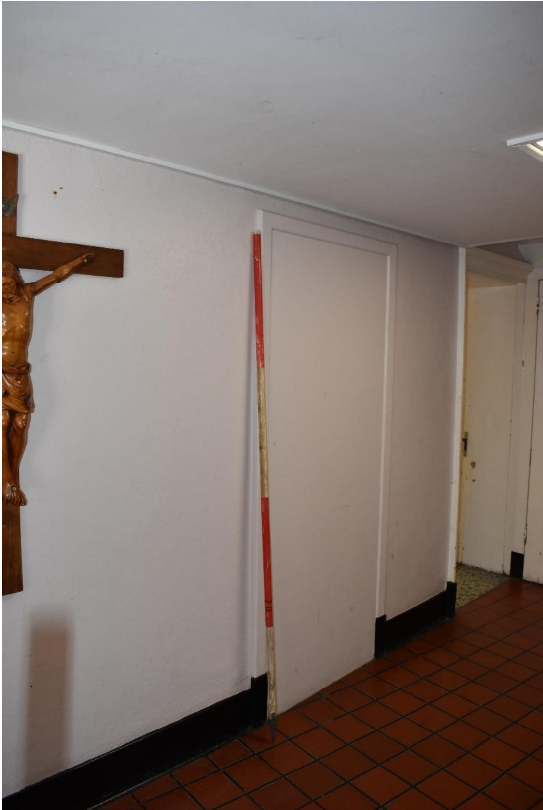
Plate 13. View of the blocked-up doorway to the easternmost office, scale 2m (looking SW)
