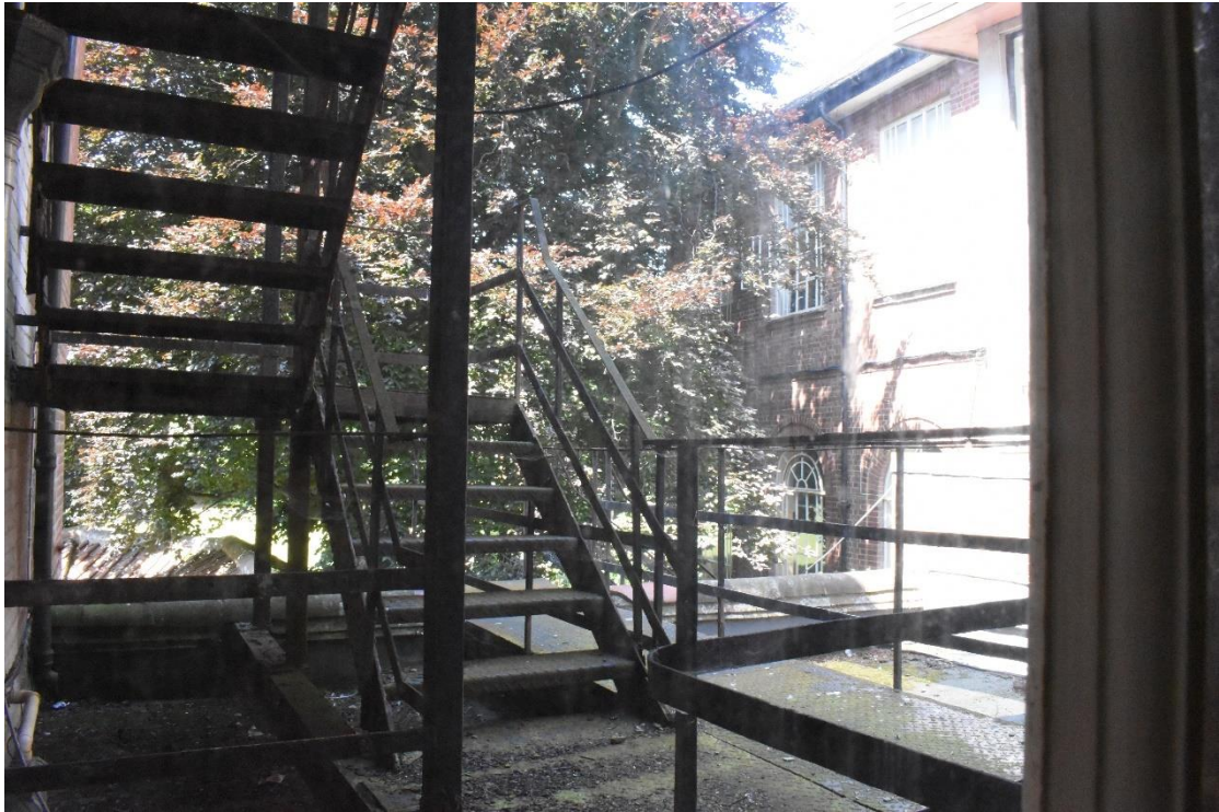
Plate 22. View of the first-floor fire escape landing (looking NW)
