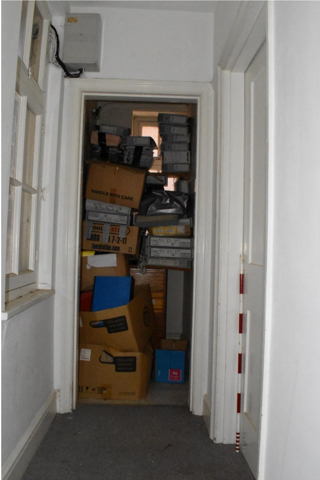
Plate 25. Internal view of the new proposed fire exit door plus the wall on the right for the store and toilet that is proposed to be moved 200m to widen the corridor, scale 1m (looking NNW)
