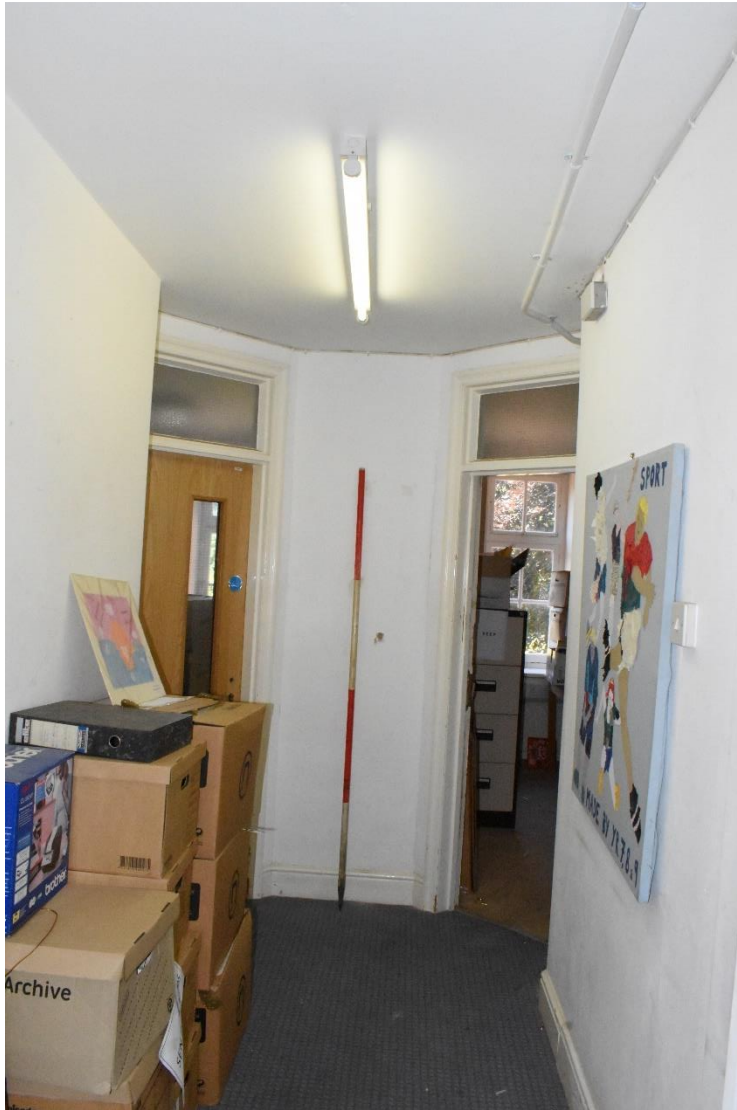
Plate 28. View of the first-floor corridor showing the two walls either side to be removed with scale showing the position where the new central wall will be built, scale 2m (looking WSW)
