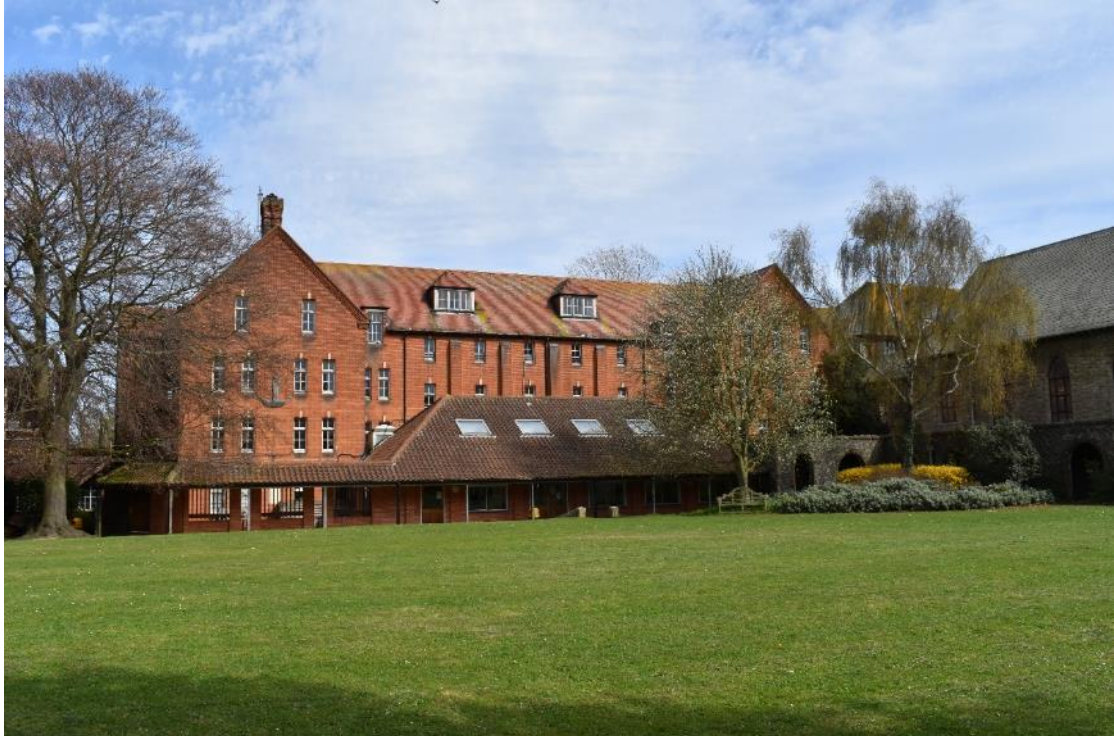
Plate 10. Front of Block C and refectory (looking E)
