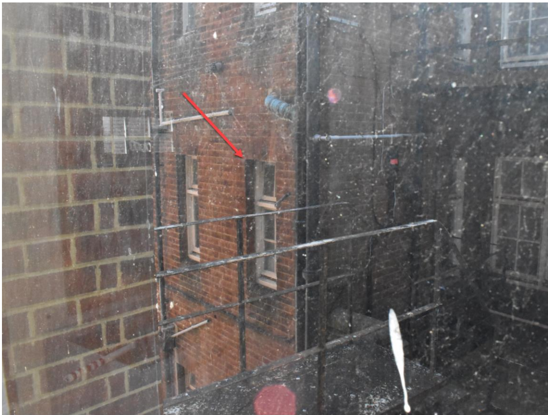
Plate 23. External view of the proposed new fire door in Block C (looking SE)
