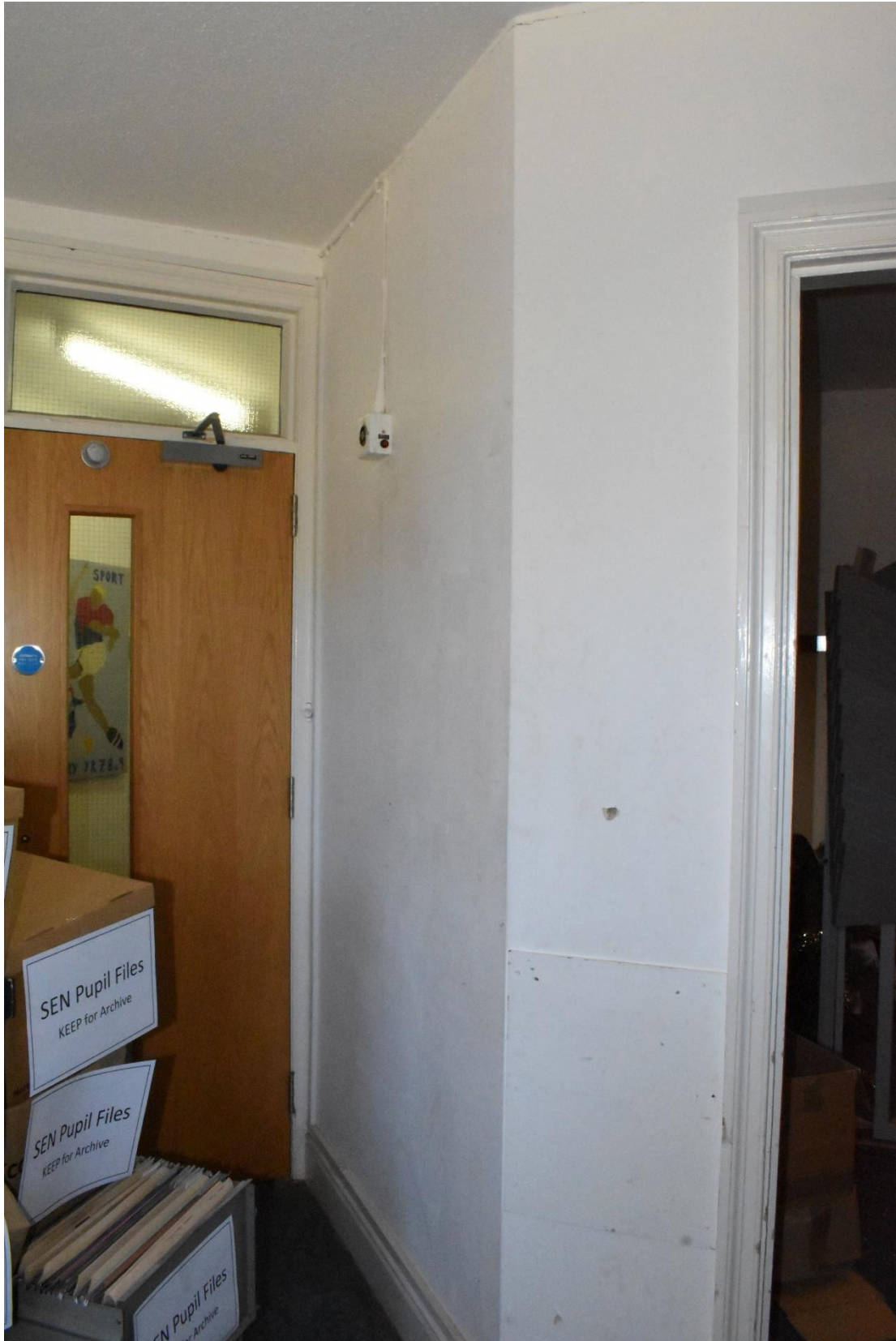
Plate 32. View of the diagonal wall and door that is proposed to be removed from the southern room (looking NE)
