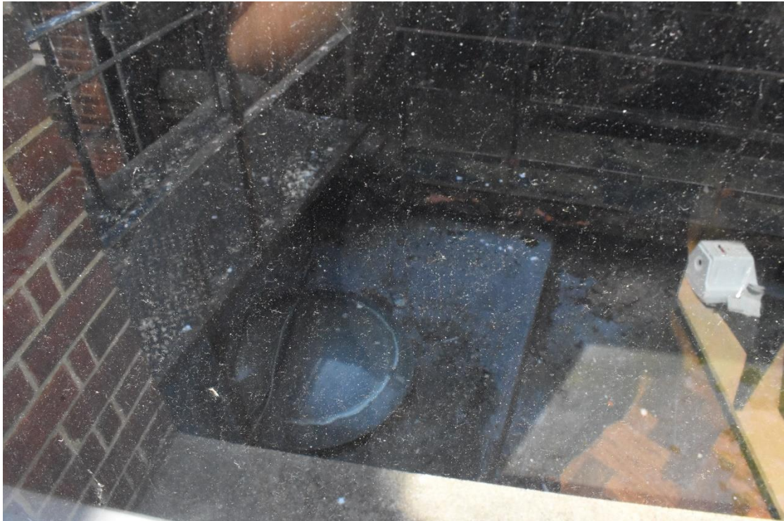
Plate 33. External view of the domed skylight that will be covered
